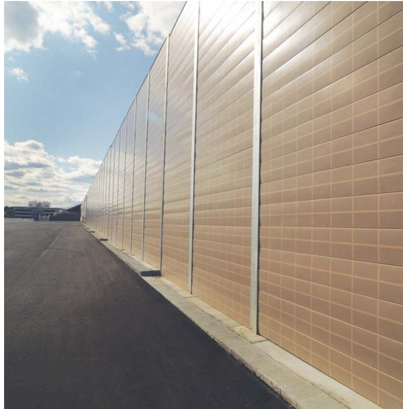
▲ Diamond Manufacturing’s Acoustax panels help reduce the noise output of this dragstrip in Concord, N.C.
